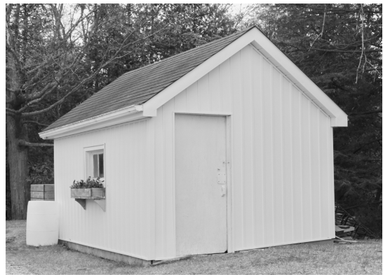
Our newly clad shed
